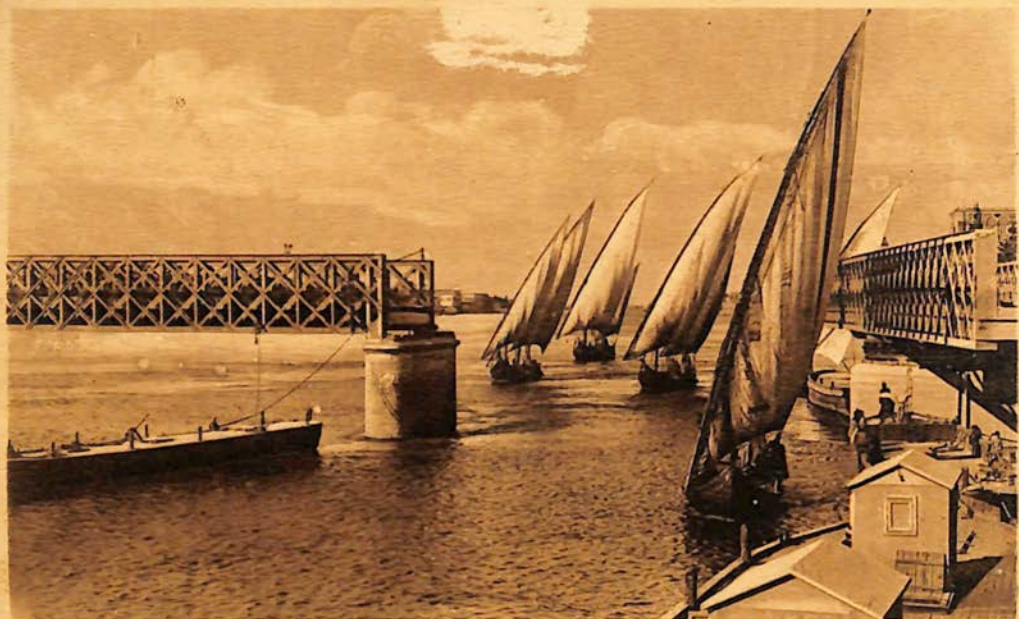
CAIRO - The Kasr-el-Nil Bridge open
