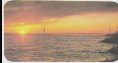
THE HUMBER BRIDGE
