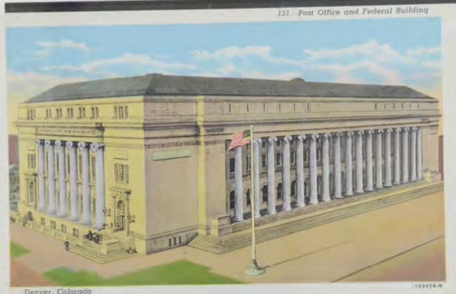
Main Post Office Building 1823 Stout Street -- Denver, Colorado
