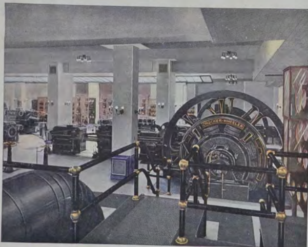
Metropolitan Life Insurance Co.'s Home Office Bldg., N.Y. City. Corner of Engine Room. Electrical and elevator equipment the largest of any office building in the world.
