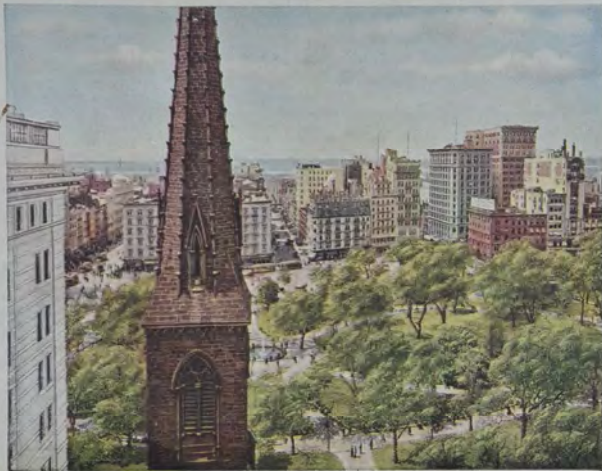
Looking west from roof of Home Office of the Metropolitan Life Insurance Company of New York, Madison Square in the foreground.
