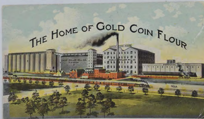
Plant of EAGLE ROLLER MILL CO., New Ulm, Minn. Daily Capacity 5,000 Barrels, Elevator Capacity 2,600,000 Bushels.
