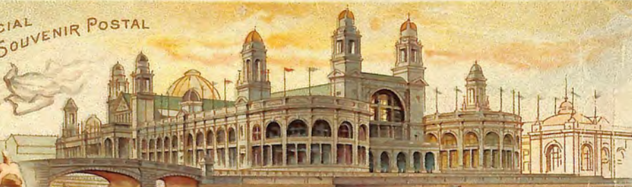
THE ELECTRICAL BUILDING.
