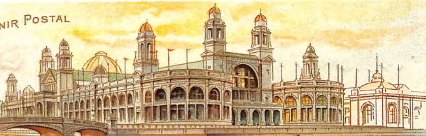
THE ELECTRICAL BUILDING.
