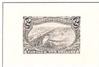
#293 Mississippi River Bridge
