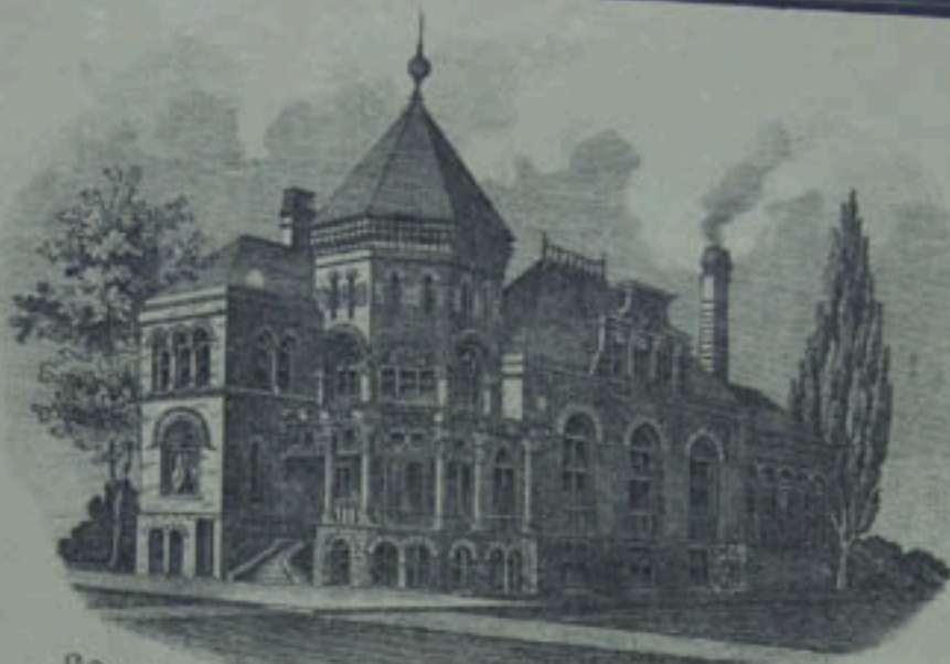
CONNECTICUT FIRE INSURANCE COMPANY BUILDING
