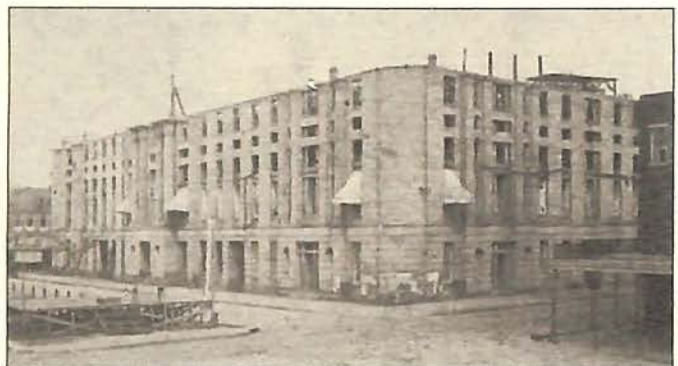
New U.S. Customs House being built 1848
