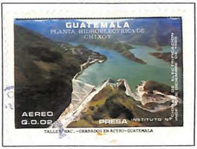
Chixoy Hydroelectric Power Plant 1987
