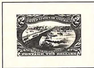
MISSISSIPPI RIVER BRIDGE AT ST. LOUIS
