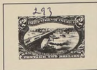
MISSISSIPPI RIVER BRIDGE AT ST. LOUIS
