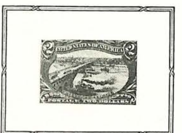
Mississippi River Bridge
