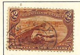
Mississippi River Bridge
