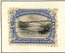
Bridge at Niagara Falls
