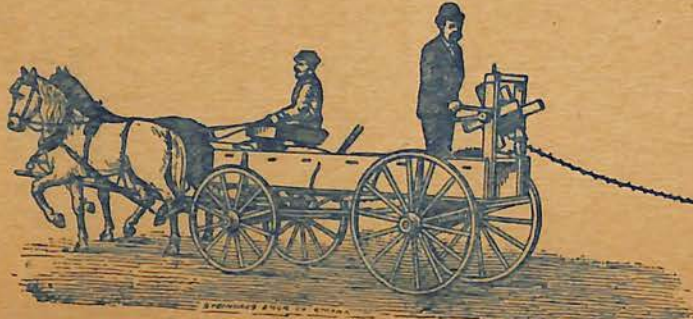
Figure 2. Putting out Barbed Wire.
