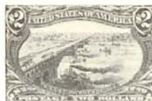
Mississippi River Bridge
