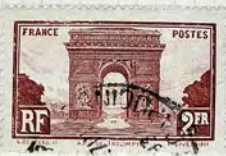
Type A. Defect in top plinth of Arch
