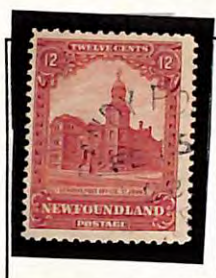
GENERAL POST OFFICE, ST. JOHN'S
