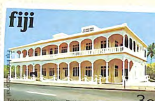
Telecommunications Building, Suva
