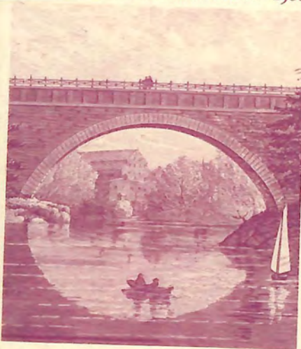
ECHO BRIDGE NEWTON UPPER FALLS (1876)
