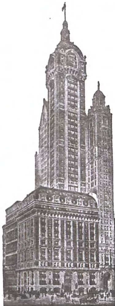
SINGER BUILDING, NEW-YORK 47 STORIES — 612 FEET HIGH
