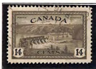
Power station, St. Maurice River
