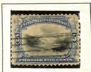
Bridge at Niagara Falls
