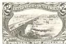
Mississippi River Bridge
